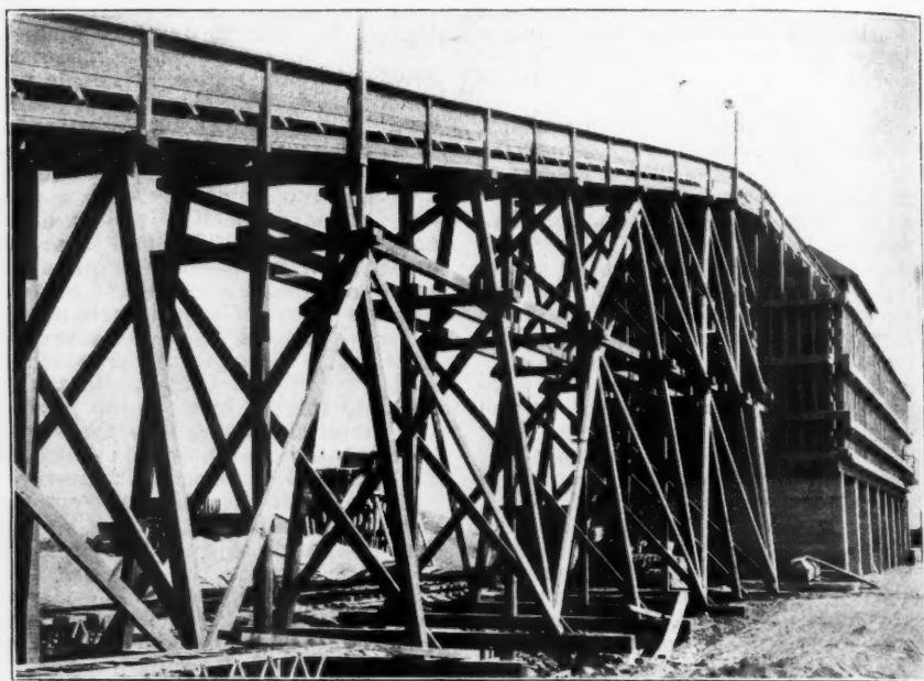
Detail of Trestle Support for Conveyor to Bins at Long Beach
